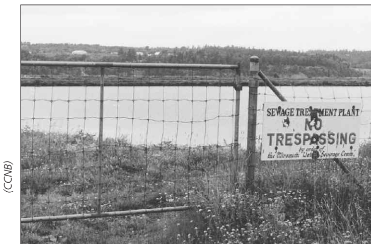
Sewage lagoons are passive treatment systems.
