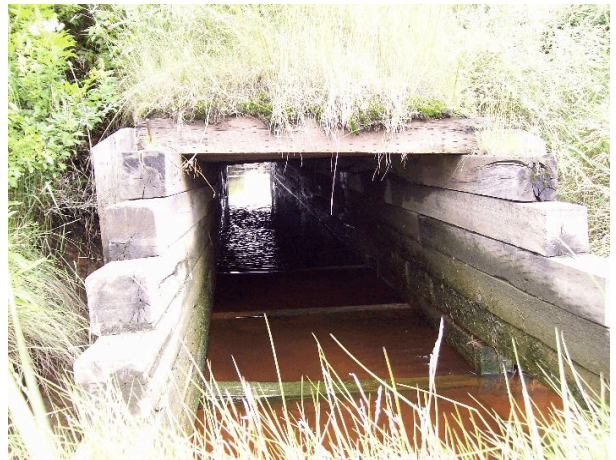
Wooden culvert in good condition (CCNB photo 2006)
