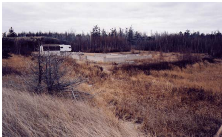
Building foundation near the edge of marsh at the end of a private road. (CCNB photo 2006)
