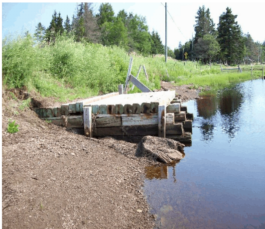
Well maintained wooden culvert (CCNB photo 2006)
