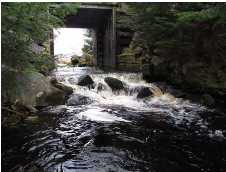
Photo 1 Barrier to Fish Passage Structure at Entrance to Nashwaak Lake.
